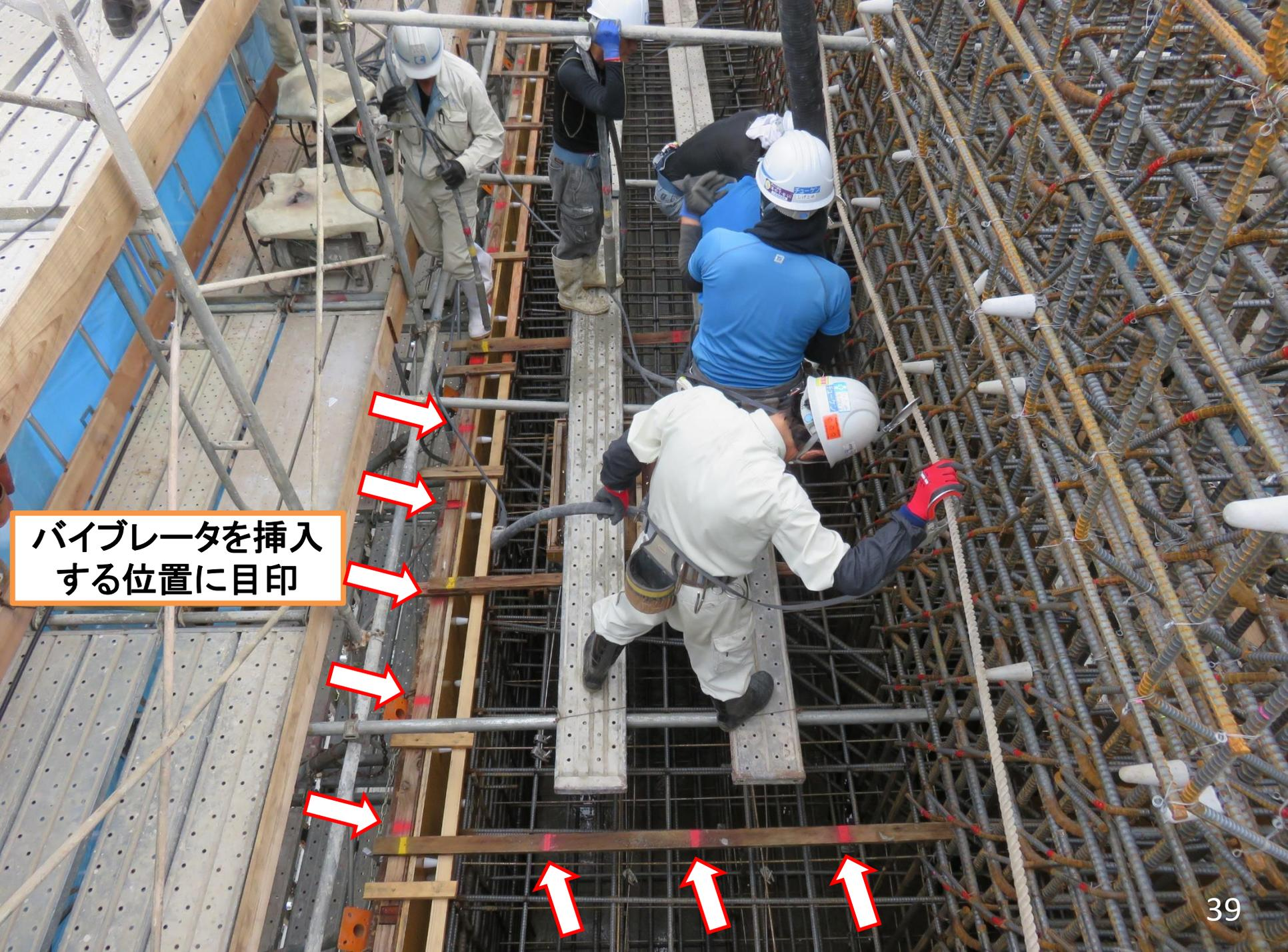
A high-angle photograph of construction workers on a steel rebar grid. The workers are wearing white and blue uniforms and hard hats. They are positioned on a narrow metal walkway. The rebar grid is dense and extends across the frame. Red arrows point to specific locations on the grid where vibration plates are to be inserted. A text box in the lower-left corner contains the text 'バイブレータを挿入する位置に目印' (Marking the position for vibration plate insertion).
